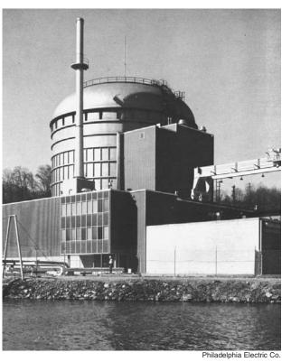
General Atomics' Peach Bottom reactor, 65 miles southwest of Philadelphia, began commercial operation in 1967. This high-temperature, graphite-moderated, helium-cooled reactor operated between 1967 and 1974 at 110-MWt, using highly enriched uranium with thorium.
